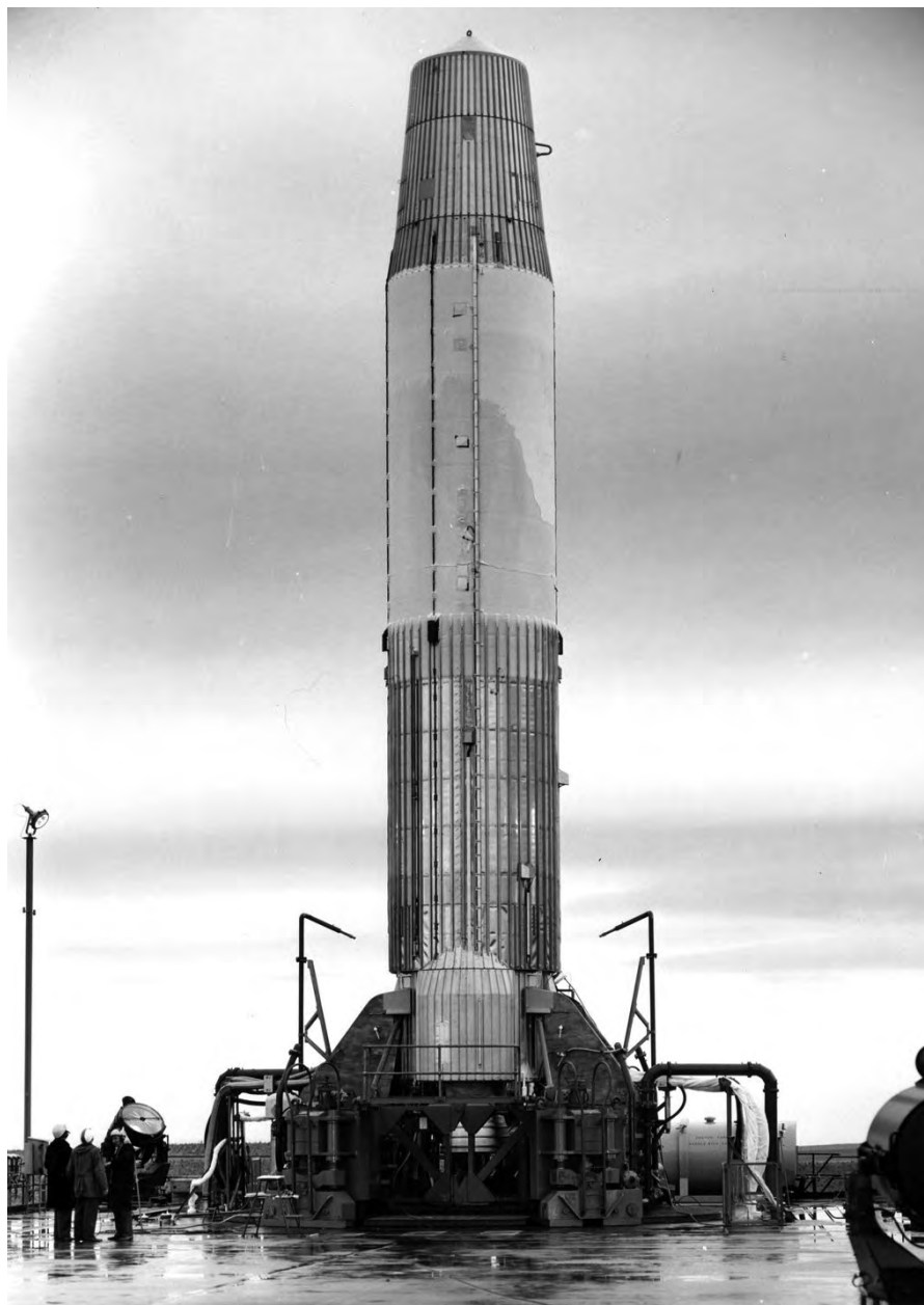
Britain's Blue Streak ballistic missile, designed in 1955 and tested at Woomera test range, Australia. It was used as the first-stage of the European satellite launcher, Europa. (Google Images)
