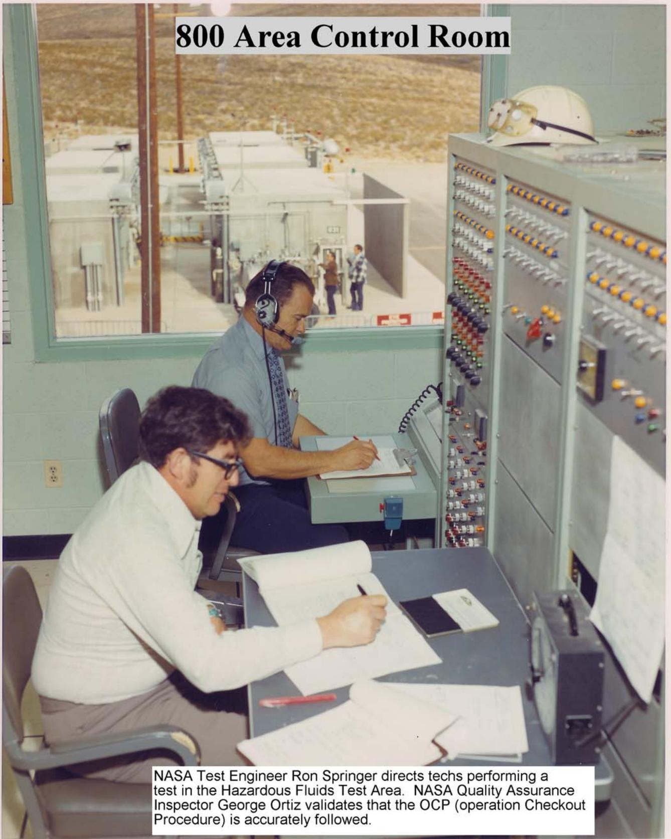
NASA Test Engineer Ron Springer directs techs performing a test in the Hazardous Fluids Test Area. NASA Quality Assurance Inspector George Ortiz validates that the OCP (operation Checkout Procedure) is accurately followed.
