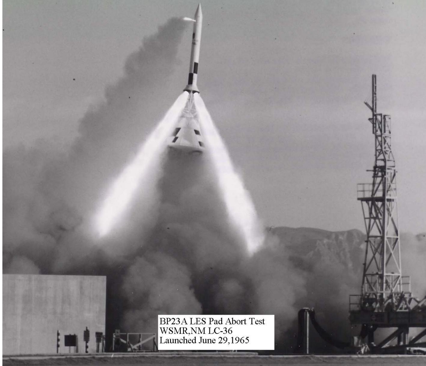
*Photo A-11 - Launch escape system's fired rocket motor just before the explosive bolts were energized.*
